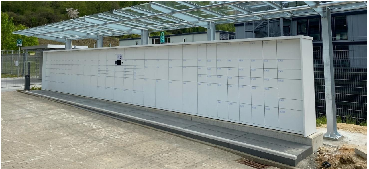
Fig. 118 Example of an outdoor parcel box system
